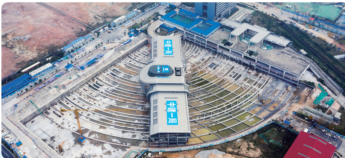
Large-scale building relocation technology and equipment
